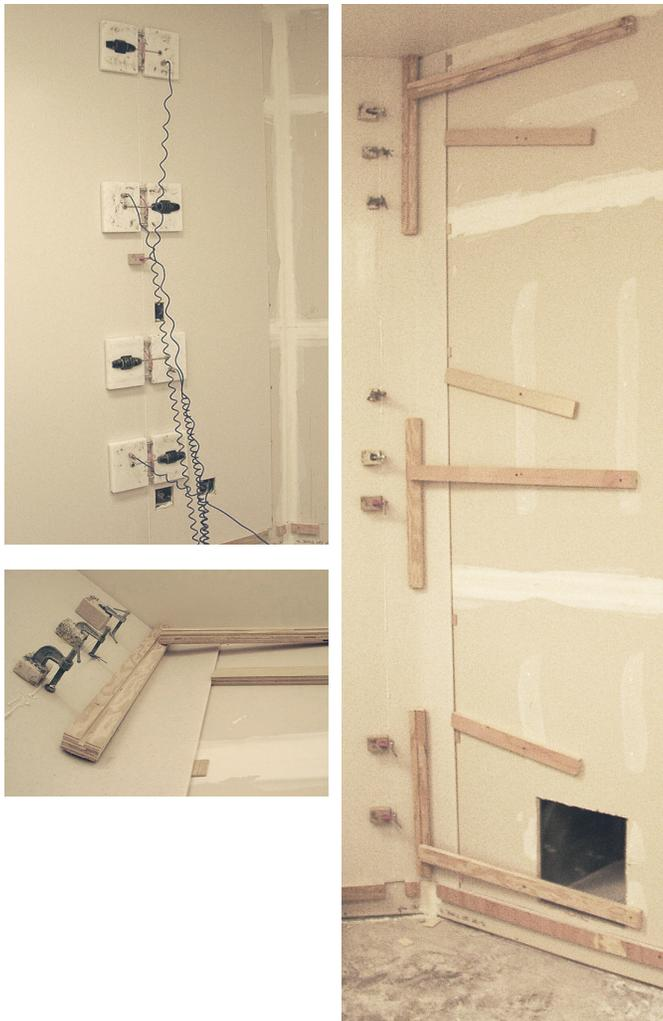
Use vacuum clamps and/or bracing to pull or push and hold seams together. Adjustment blocks can be mounted with hot melt glue to help align adjacent surfaces to achieve inconspicuous seams. Use of a wooden shim is shown in top right view to maintain silicone adherent thickness. Figure P-2 shows the assembly of a tongue and groove seam for 6 mm (1/4") solid surface sheet.
